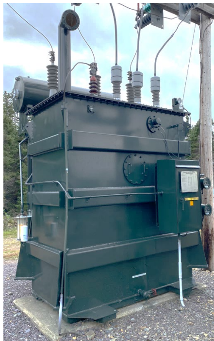
Figure A-6: SMV-T1 Power Transformer
