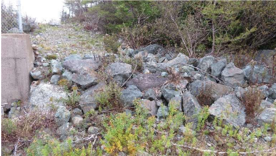
Figure 2 – Abutment Riprap
