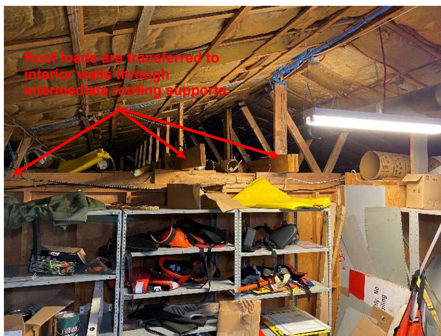
Figure 2: Roofing System
