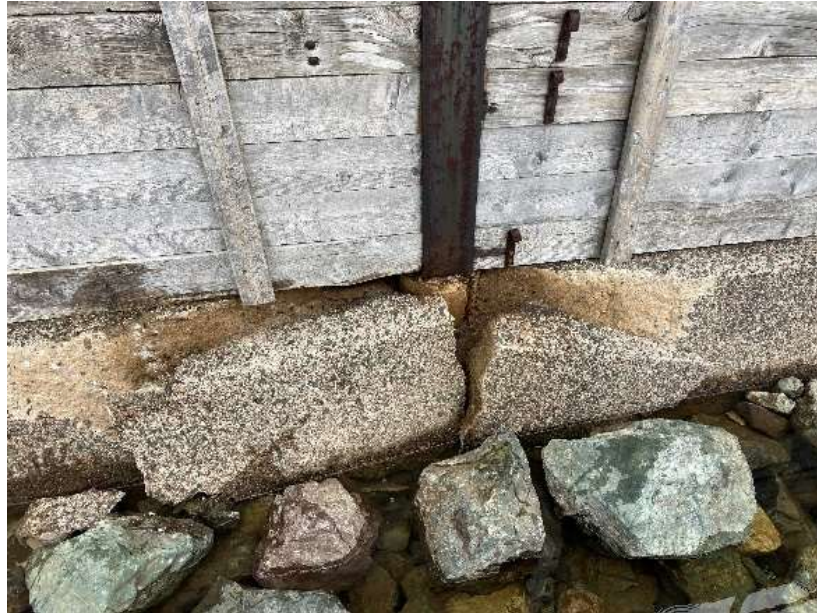
Figure 8 – Foundation Damage
