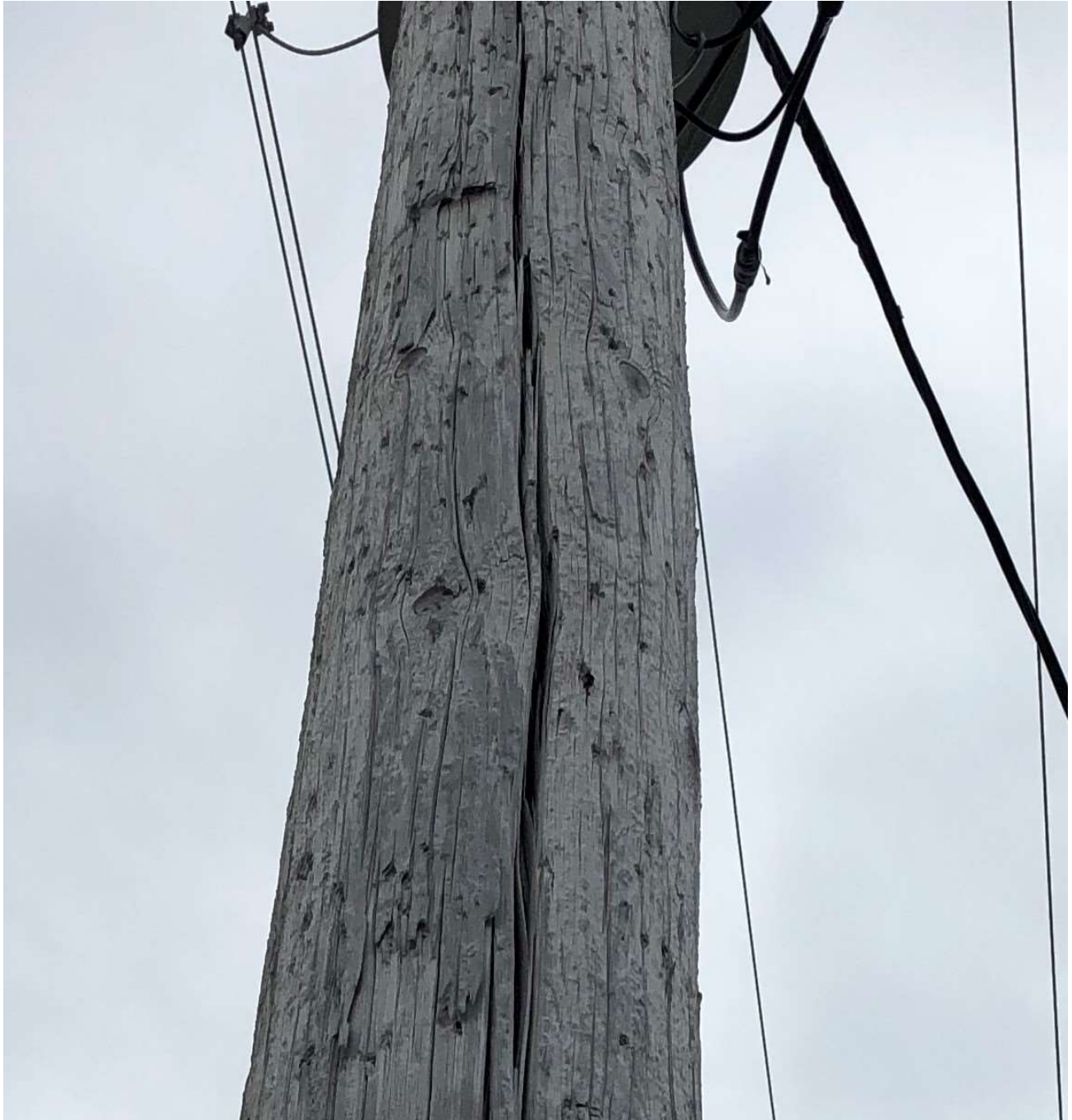
Figure A-2: Hollow Pole, Large Splits
