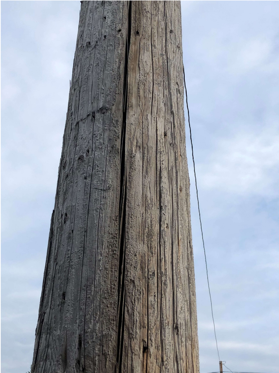
Figure A-3: Deep Splits, Hollow Pole
